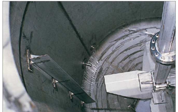
Tank sampling valve Inside of vessel
